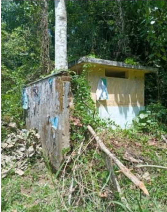
Figure 08: Abandoned toilet system
